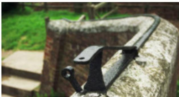
**Figure 2 - The roller is lost but the guard iron remains in situ on this bridge parapet**
